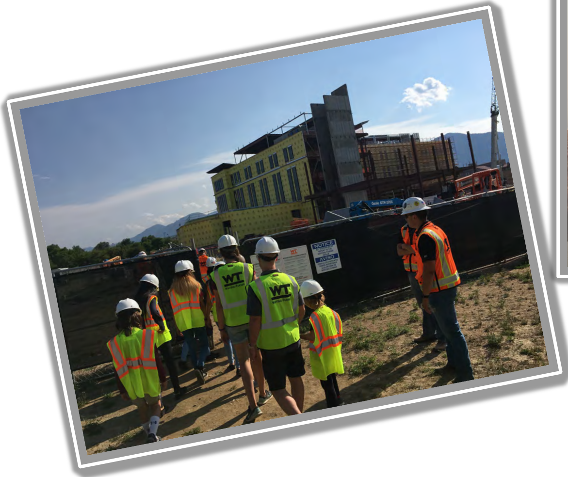
Construction Site Tour
